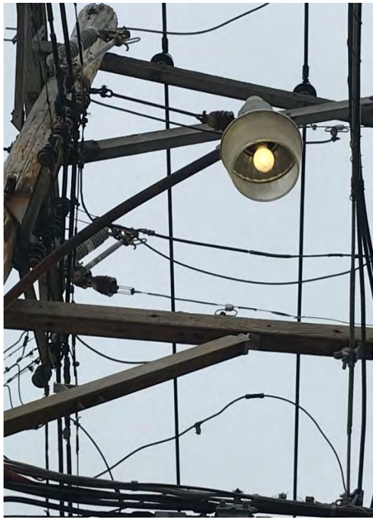
100W Mercury Vapor Alley Light Fixture
