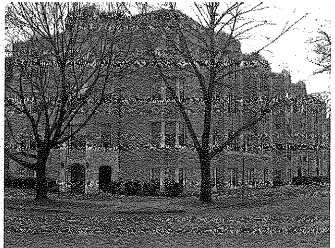
Figure 89: Apartments at 225-227 N. Grove (1928), designed by Dubin & Isenberg.
