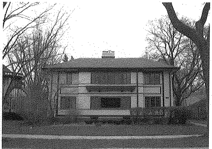
Figure 56: E.P. Ward House (1915), 724 Linden Avenue.
