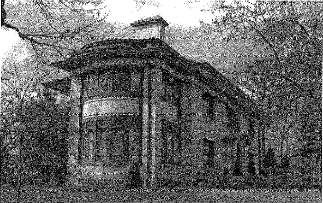
Figure 66: James Hall Taylor House (1912), 405 N. Euclid Avenue.
