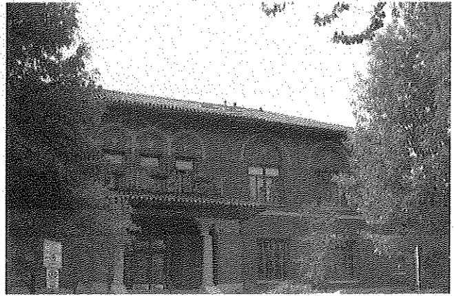
Figure 94: Oak Park Club (1923), 721 Ontario Street, designed by Holmes & Flinn.
