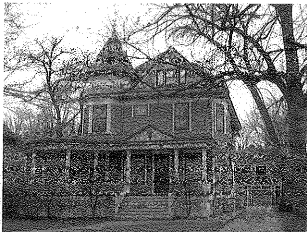
Figure 12: F.E. Hoover House, (1896) at 521 N. Euclid Avenue, designed by Eben E. Roberts.
