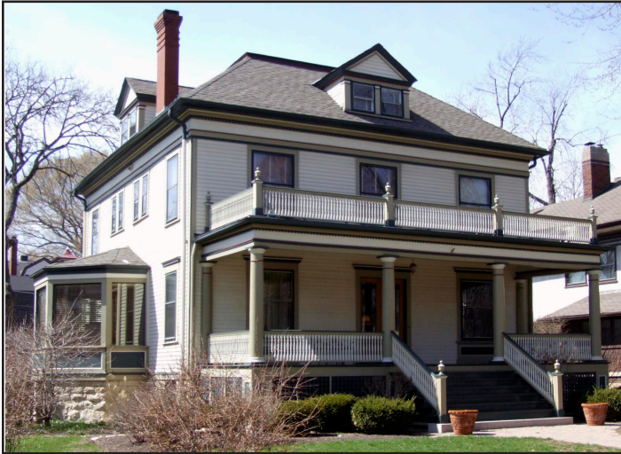
The Award acknowledges the restoration of the house following a fire.
