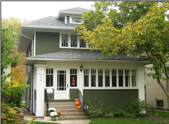
The Award acknowledges the restoration of historic wood windows and siding, and sensitive dormer additions.
