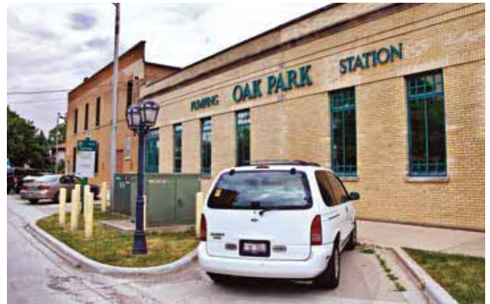
Main Pumping Station in Oak Park. Source: Jim Watkins.
