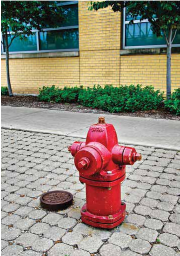
Fire hydrant in Oak Park. Source: Jim Watkins.
