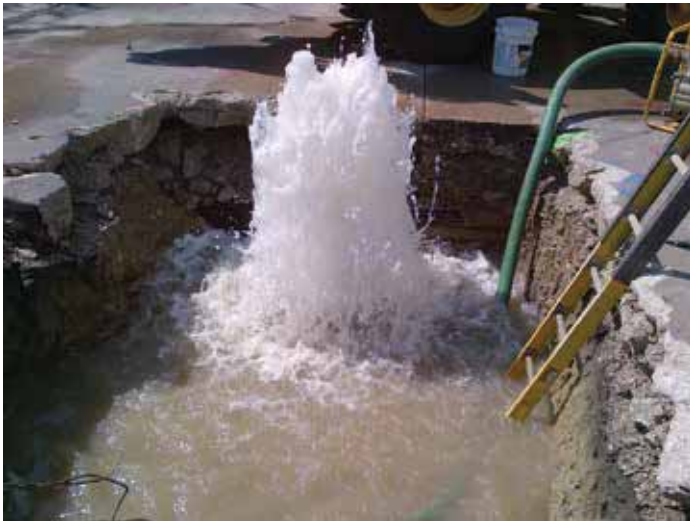
Aging Infrastructure; Oak Park water main break on a 20-inch water main. Source: Oak Park.
