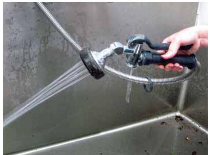
Pre-rinse spray valve. Image source: CMAP staff.
