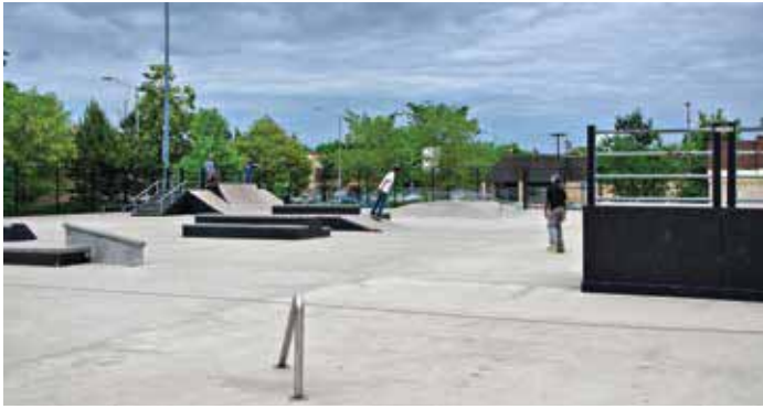
Oak Park's newest reservoir was built underneath the skateboard facilities at Stevenson Park in 2004. The additional 2.5 million gallon reservoir helped Oak Park meet the Illinois Environmental Protection Agency's required storage capacity. Source: Jim Watkins.
